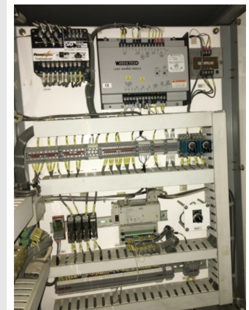
PLC PANEL WITH WOODWARD SPMA SYNCHRONIZER
